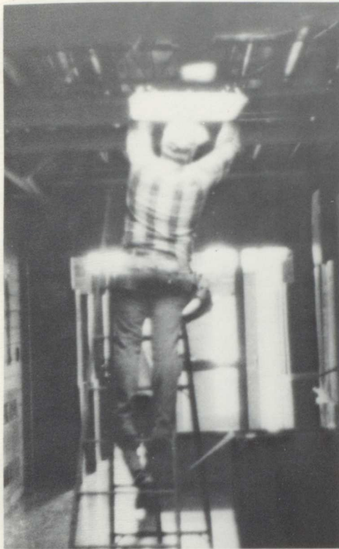
A worker replaces some of the high school ceiling.
